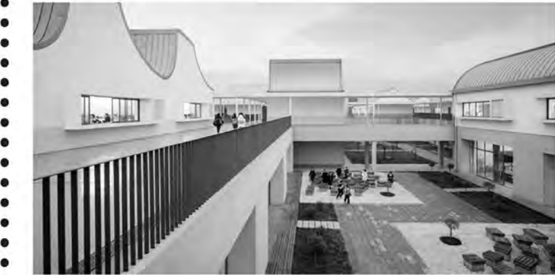
Elementary School China TAO Architecture | 2022
