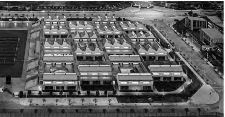
Elementary School China TAO Architecture | 2022
