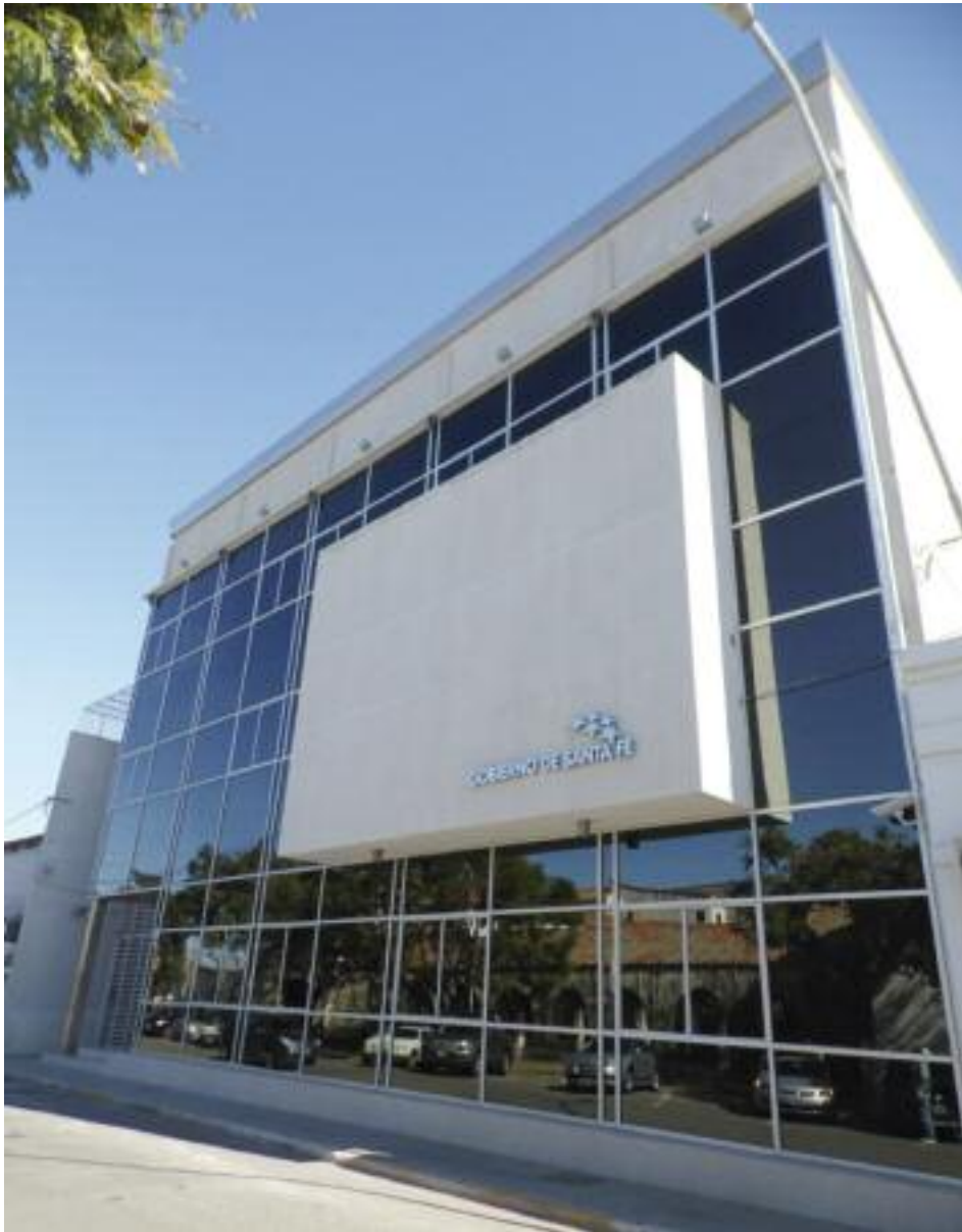
Datacenter Santa Fe
