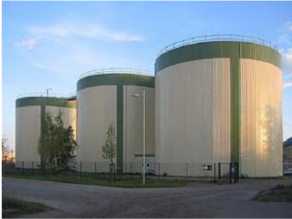
Figura 2-4: Biodigestor CSTR [15].
