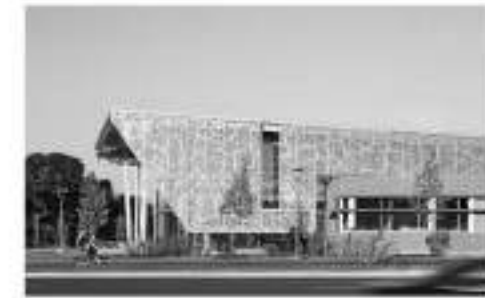
Route 9 Library Perkins and Will 2017 / EE.UU
