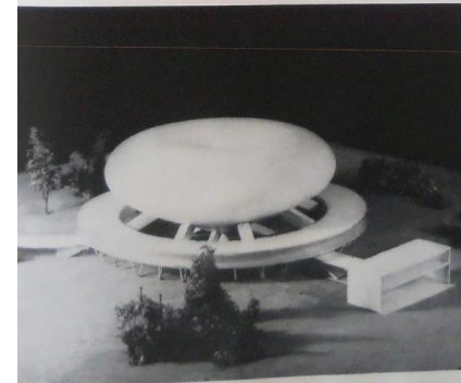
Fig. 148, left and above, project for a concert hall in which the structural shape, developed from requirements of vision and acoustics, takes on a form very much akin to that of the Horton-spheroids. (Architect: Amosce Williams.)
