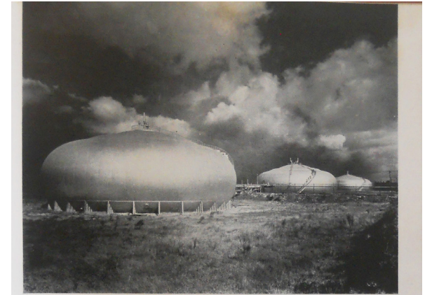
Fig. 147, above, shell construction in stiffened welded sheet steel of the 127 ft. diameter Horton-spheroid fuel tanks (80,000 bbl.) in northern Texas, provides a complete three-dimensional space-enclosing structure.
