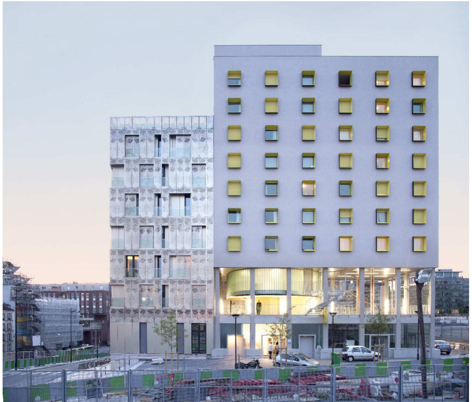
Imagen 78: Fachada. Fuente: https://www.designboom.com/architecture/stephane-maupin-elevates-dorm-on-stilts-like-a-pink-flamingo/
