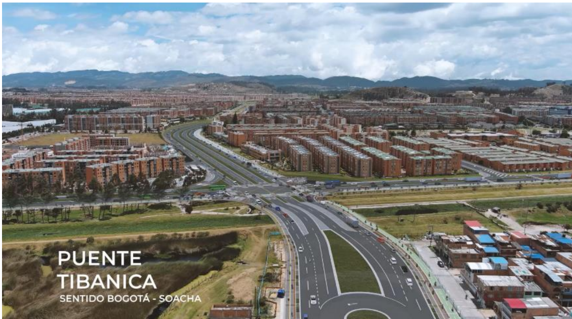
Puente Tibanica sentido Bogotá-Soacha
