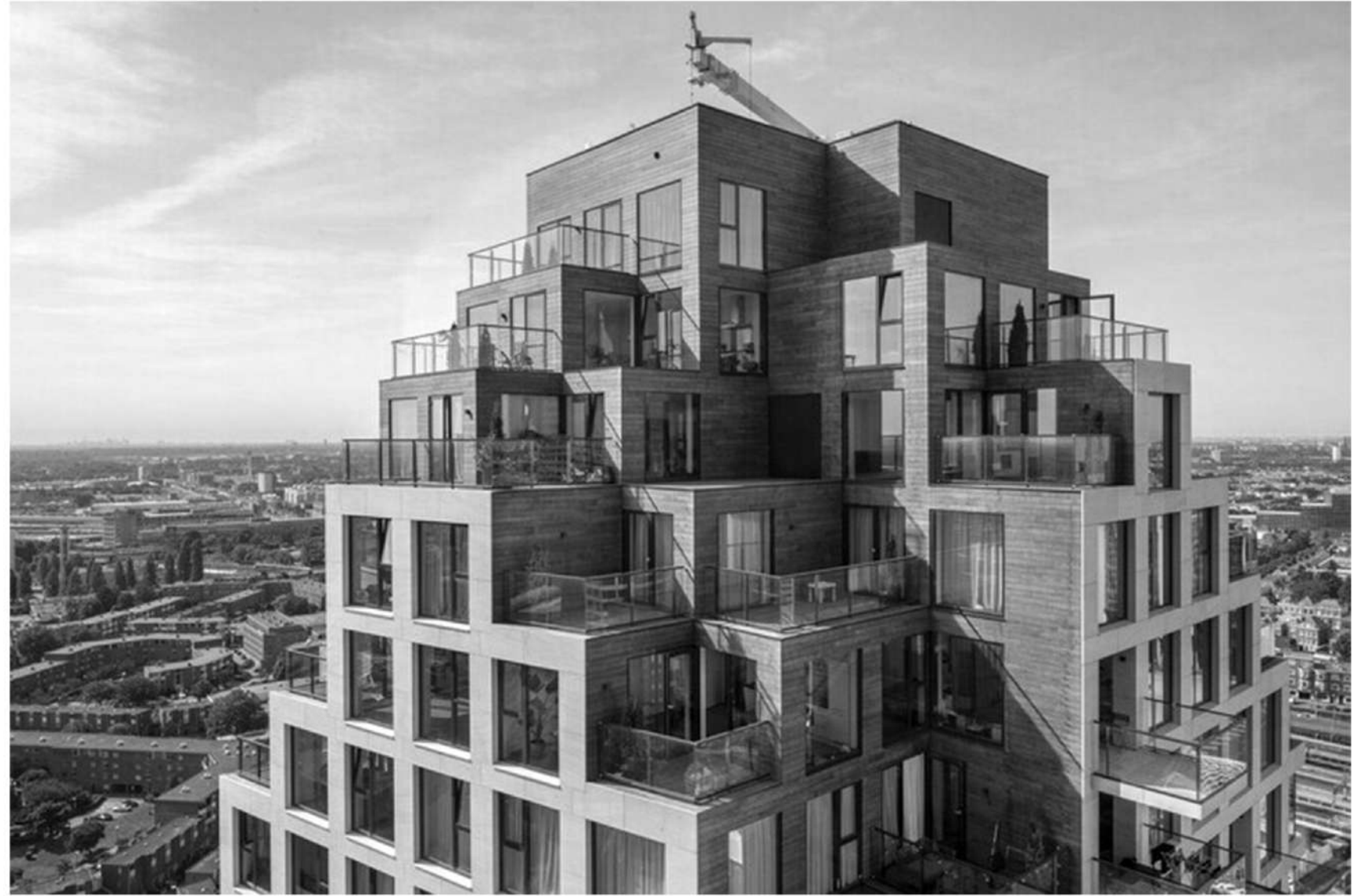
Balcones terrazas - Grotius Towers
